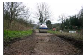
▲ Contractors create the new surface and compact it with rollers
